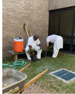
RLW: Mr. Kendrick's Landscape Construction and Design class planted shrubs at the Central Office.
