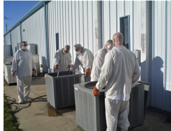
EARU's HVAC students inspecting and cleaning AC condensing units at the
