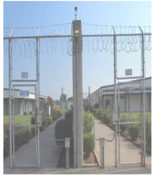
Hawkins Entry Gates
