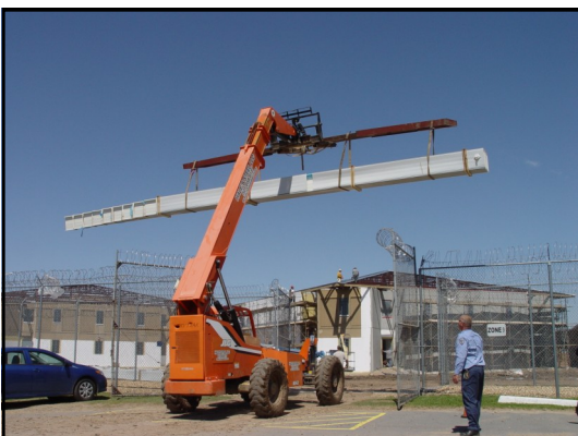
A skyhook rolls through the gates at Tucker with roof sheeting for pod renovations.
