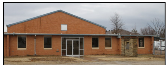
An armory built in Springdale in 1947 was renovated and became the new home for the Northwest Arkansas Work Release Center.
