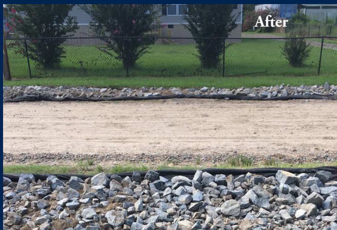
Varner Unit – Spread River Rock on Side of Road at the Pendleton Bridge - July 28
