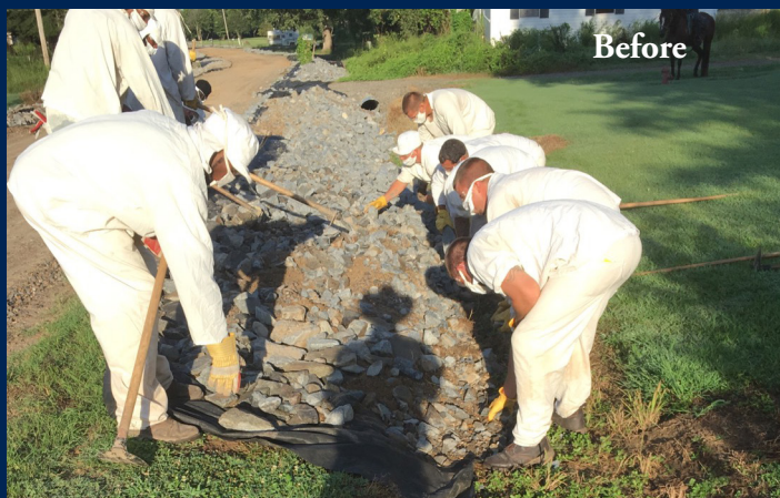
Varner Unit – Spread River Rock on Side of Road at the Pendleton Bridge - July 28
