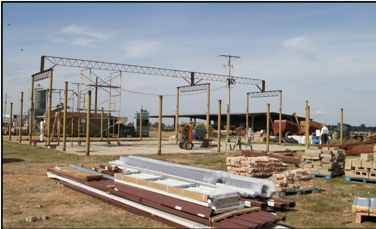
The Tucker Unit Pole Barn/Storage Shed was severely damaged by a 2012 storm, pictured below. The rebuilding, left, is utilizing salvaged material.
