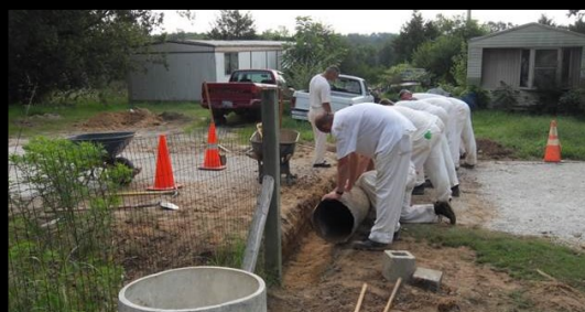
Replacing a Culvert
